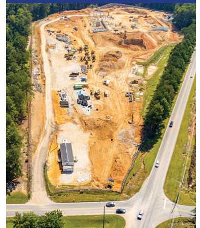
Site of Legacy Arena on Hwy. 5 at Gurley Road (October 2022 photo)
